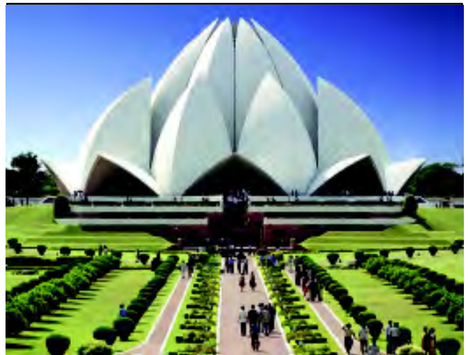
"Quality in Construction" - new mantra for construction companies in India.
